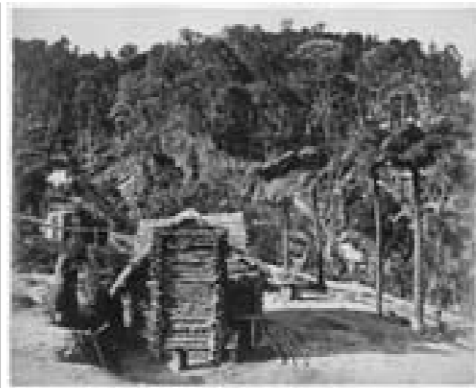
[An example of punga construction.] Daniel Louis Mundy, A digger's whare, Punga Flat, Thames goldfields, 1867-1869. Auckland War Memorial Museum. C17269.
